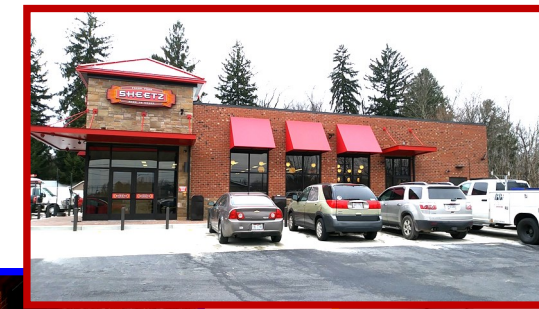
Jobsite Manager: Don King Project Manager: Jon Locketti
