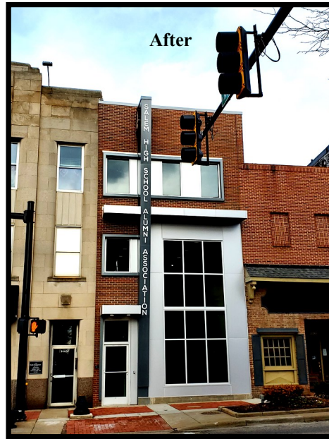
Jobsite Manager: Matt Shelby Project Manager: Jon Locketti
